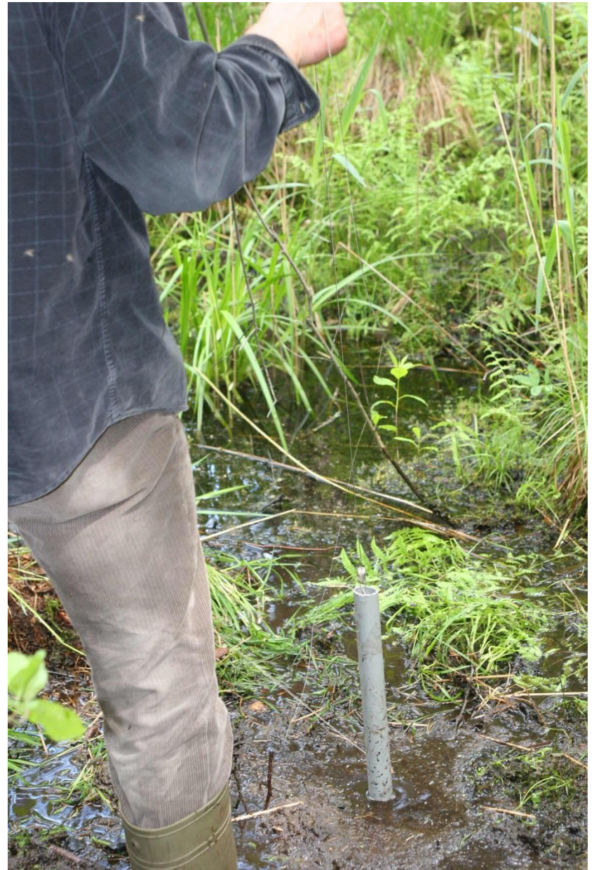
Instalation of piezometer in the Red Bog area
