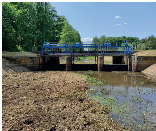
↑ Weirs in Nowa Dąbrowa (centre of the Kampinos Forest) and in Sianno (west of the forest). The former, thanks to the renovation recently carried out by PGW Wody Polskie [National Water Management Authority], is the only well-performing weir in the Forest. The latter, due to its leakage and late closure after winter, is unable to hold water during dry periods. (photo: Michał Miazga, Anna Andrzejewska)
