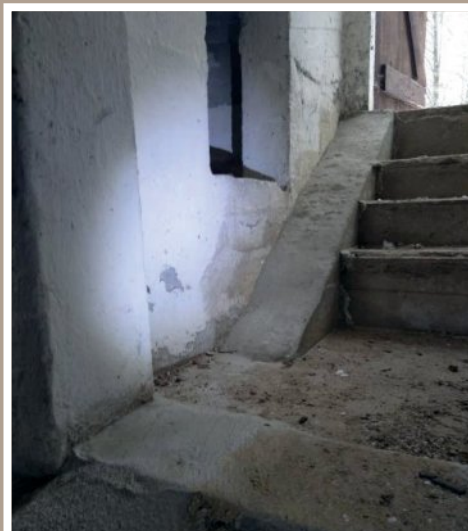
↑ A ramp helping amphibians leave their wintering site in a root cellar, a remnant of one of the former Kampinos villages. (photo: Karol Kaszyński)
